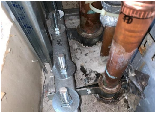
Figure 1: Newly installed and designed anchors.
